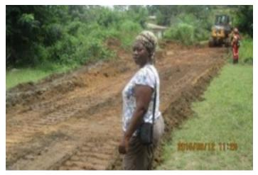
The end result was a fine road from the new highway into the school, a distance of about half a mile. The contractor crowned and graded the road to provide drainage in the rainy season. Although the rain slowed work somewhat, using heavy machinery the project took only three days.
